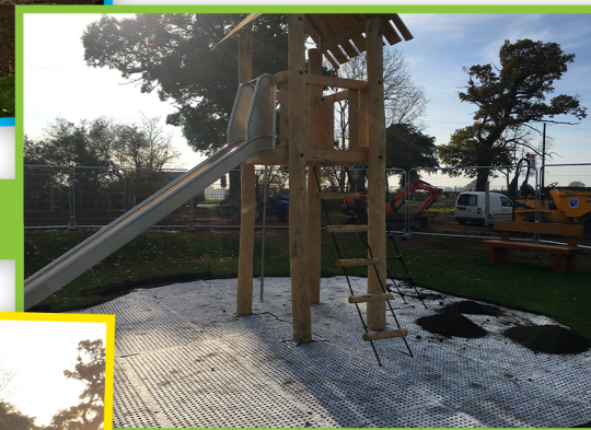
Install SmartPlay shock pad
